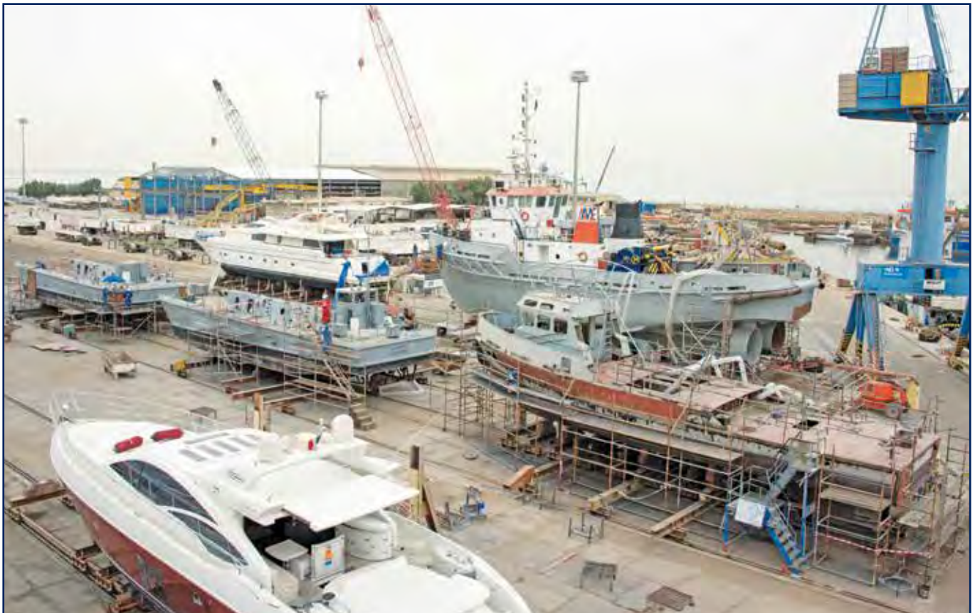
Dry-Docking and Repair of Various Vessels at the Repair Bays
