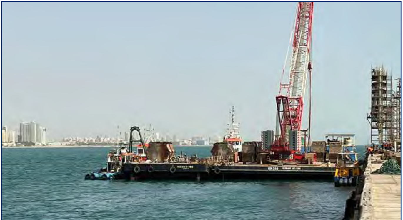
Work Barge for Marine Maintenance Works at Mina Al Ahmadi Refinery
