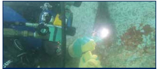
Professional Diving Services - Underwater Welding
