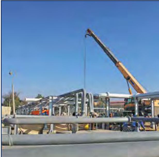
Piping Works at Water Facility Upgrade Project for Kuwait Oil Company
