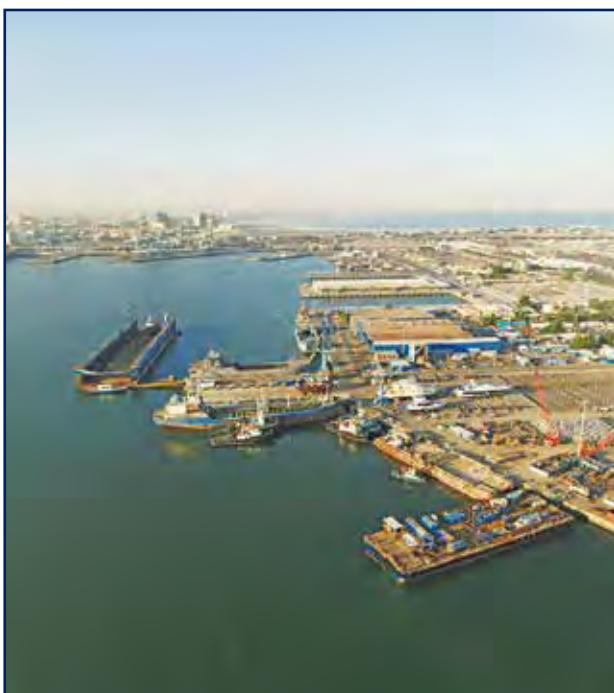
Aerial Overview of Shipyards
