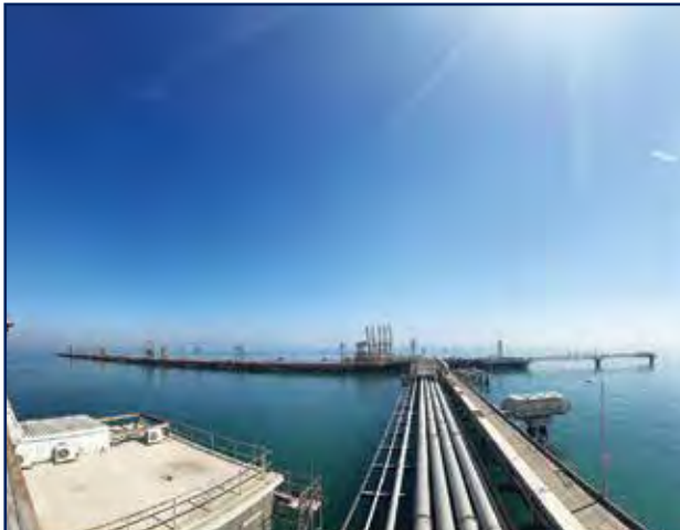
Enhancement of North Pier Integrity for Kuwait National Petroleum Company
