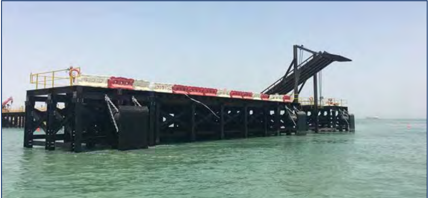
Construction of Temporary Offloading Jetty at Ras Al Ardh Logistics Station
