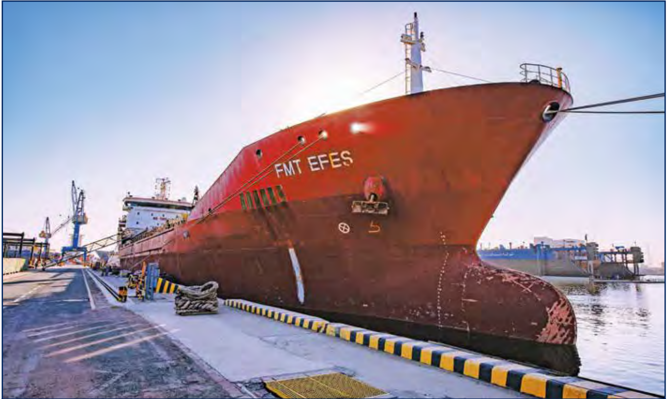
Alongside Repairs of Various Vessels for Local and International Clients
