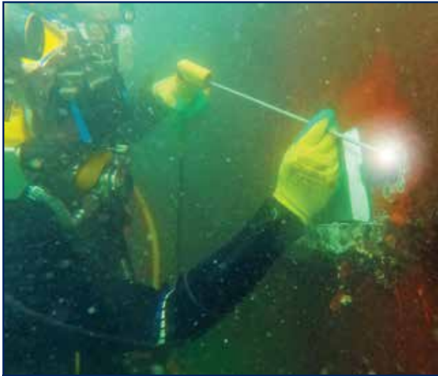
Professional Diving Services - Underwater Welding
