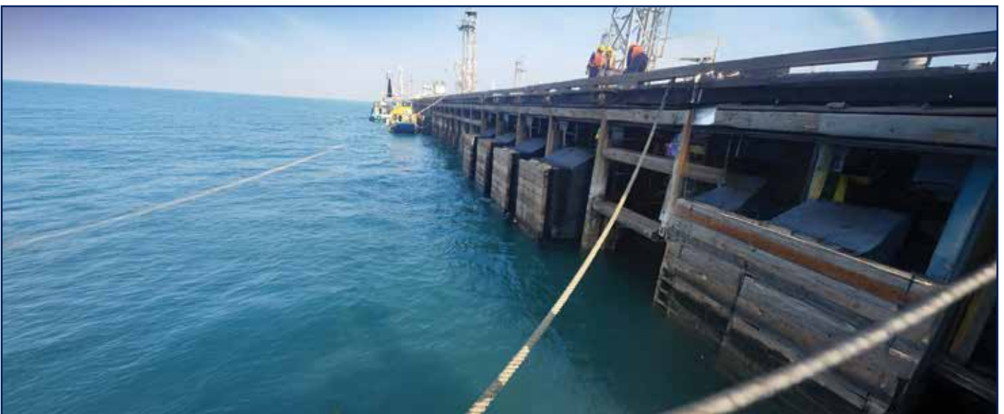
Marine Maintenance Works at Mina Al-Ahmadi Refinery for Kuwait National Petroleum Company
