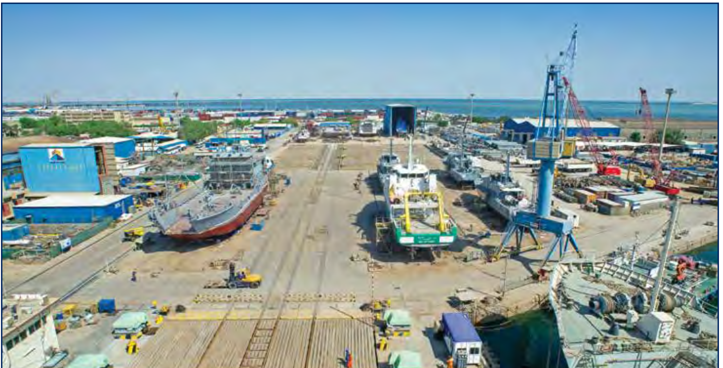
Dry-Docking and Repair of Various Vessels at the Repair Bays
