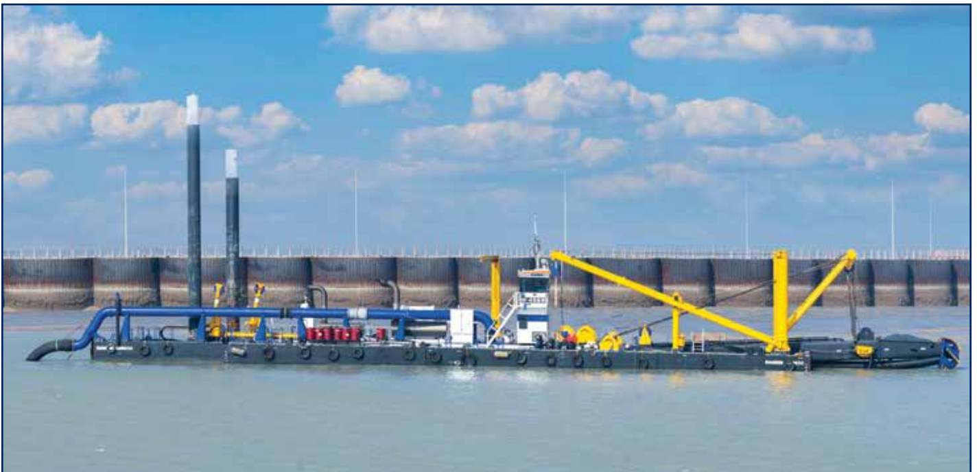
Cutter Suction Dredger
