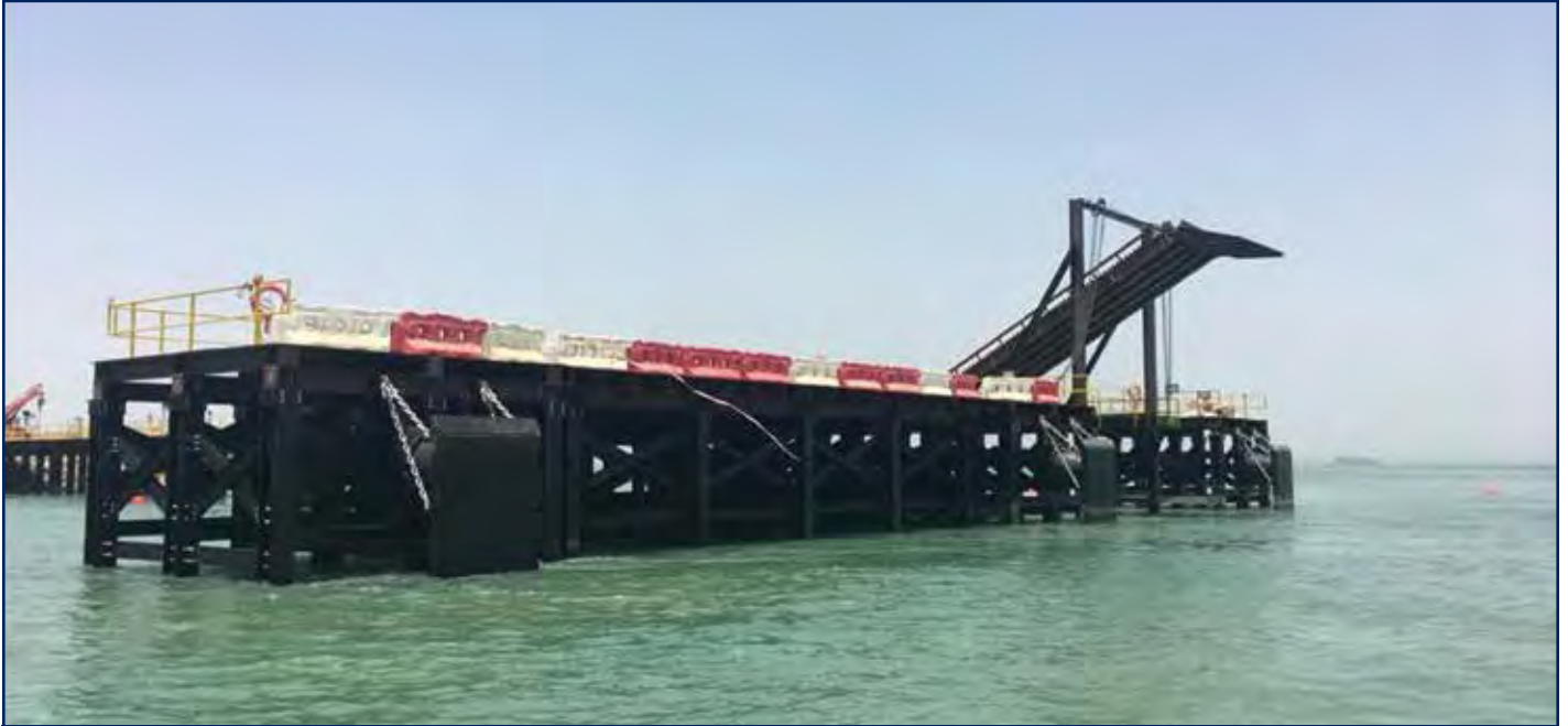
Construction of Temporary Offloading Jetty at Ras Al Ardh Logistics Station
