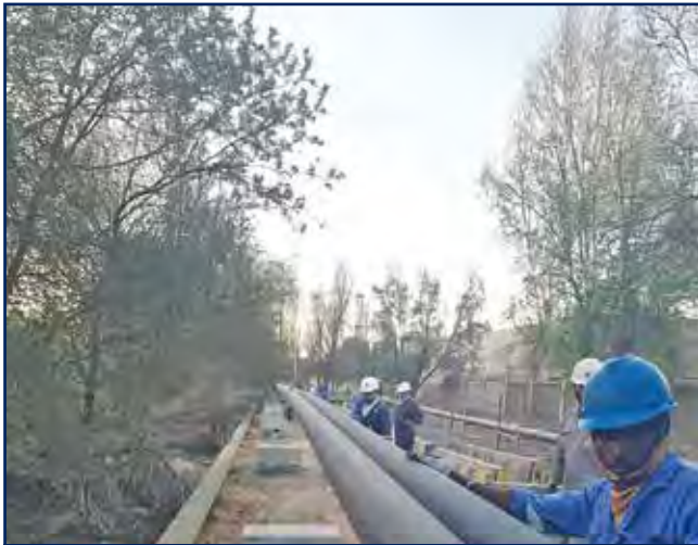
Pipeline Construction for the Supply of Nitrogen for KNPC Refineries
