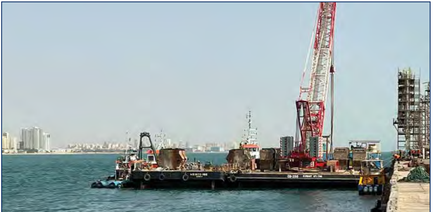
Work Barge for Marine Maintenance Works at Mina Al Ahmadi Refinery
