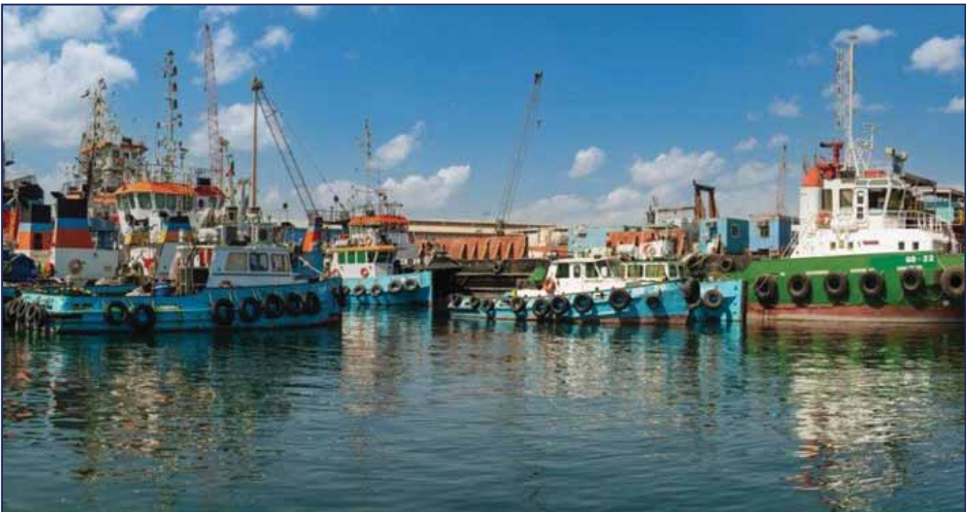
Berthing Facilities at Shuwaikh Port
