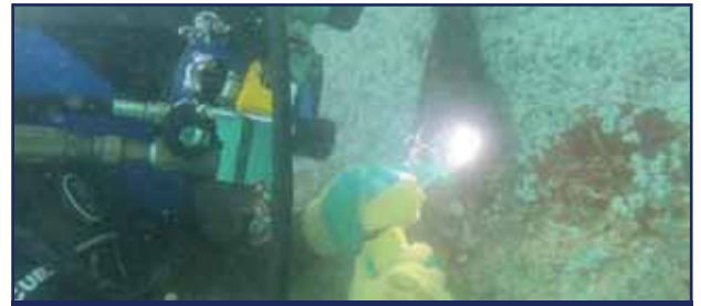
Professional Diving Services - Underwater Welding
