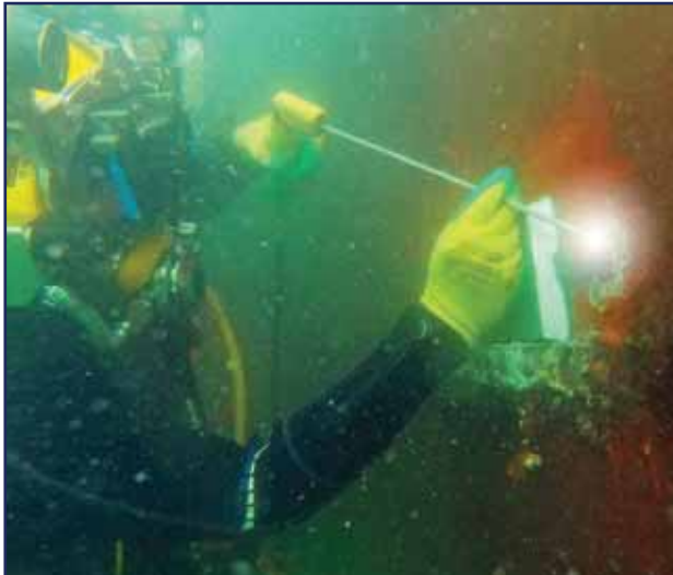
Professional Diving Services - Underwater Welding
