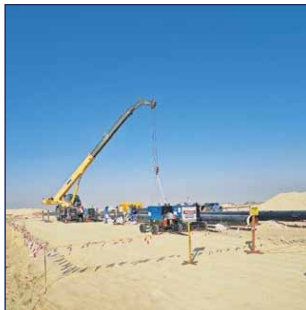
Pipe Welding Works at Gas Condensate Network Project for Kuwait Oil Company
