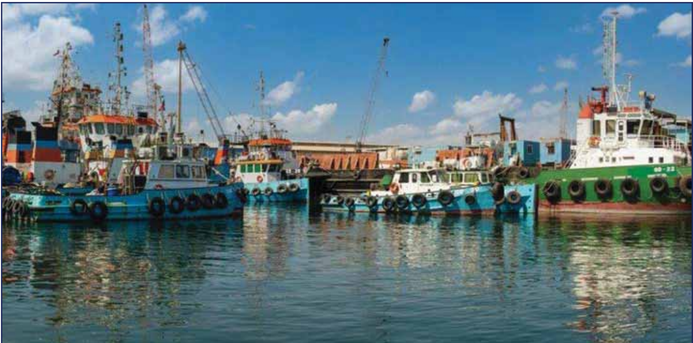
Berthing Facilities at Shuwaikh Port
