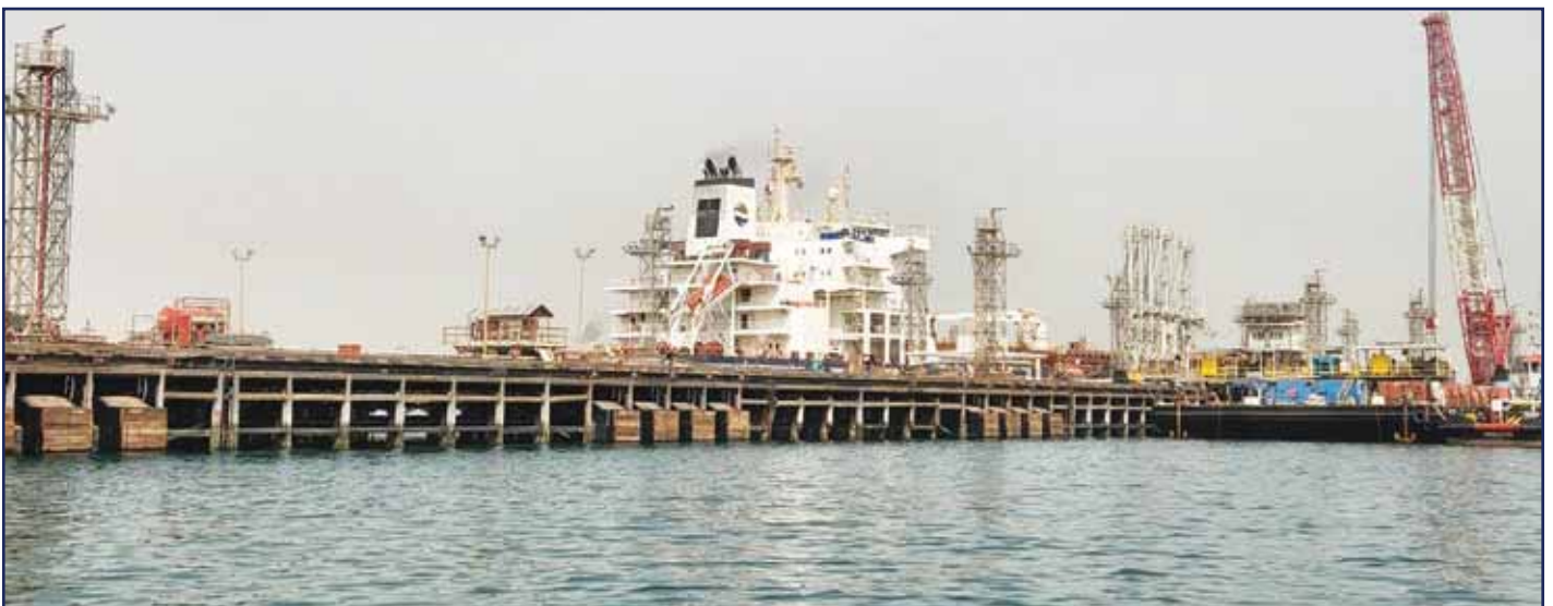
Marine Maintenance Works at MAA Refinery
