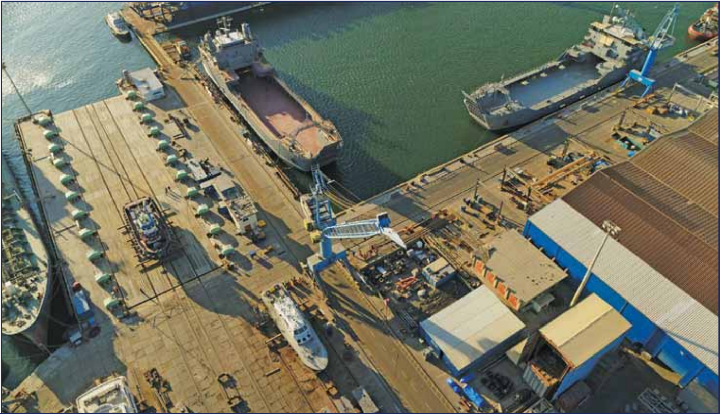
Aerial Overview of Syncrolift & Jetties
